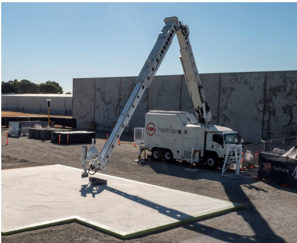
The building of an 'F' structure in progress. The two-course F structure comprises every block configuration and combination required for the build of a full home structure.
