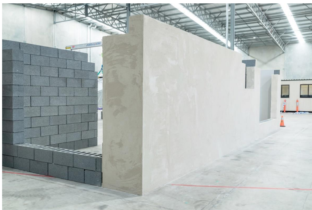
The finished three-bedroom, two-bathroom structure built at FBR's test facility with the Hadrian X in under three days
